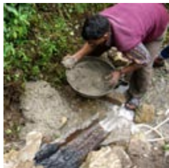
S--- building the platform
